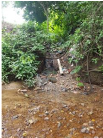
Figure 7. Grey water discharge pipe.
