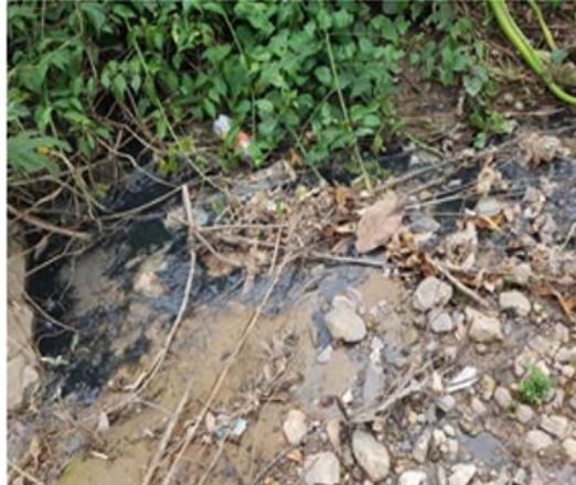
Figure 8. Grey water discharge pipe
