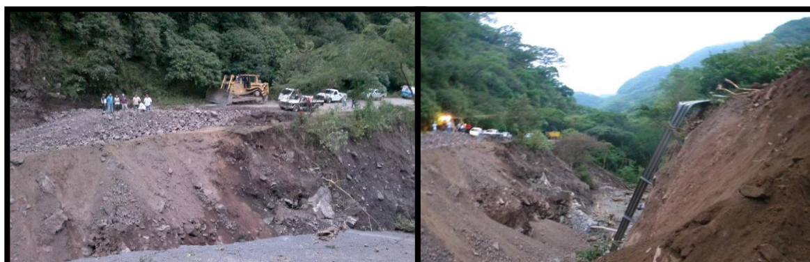
Figure 11. Damage caused by hurricane “Jova” on communication routes.
