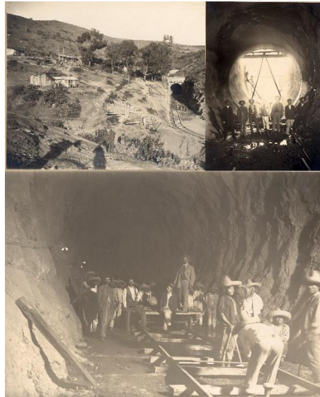
Figure 6. Construction of the Porfirio Díaz tunnel, commonly known as El Coajín
